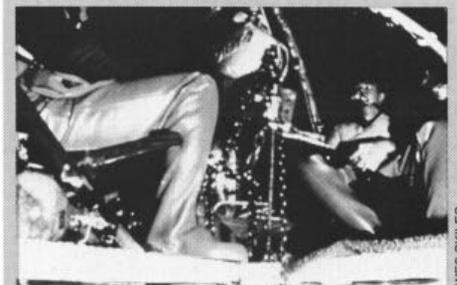
Cover: The decompression habitat used at the Wakulla Springs Project, 1987. The variable-depth habitat was capable of housing six divers and could be manually raised by the dive team during ascent.
